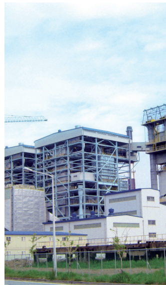
Power Plant Boiler
