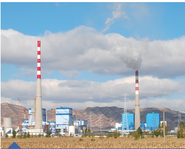
Shanxi Datang International Yungang Thermal Power Exhaust Steam Waste Heat Recovery Project
